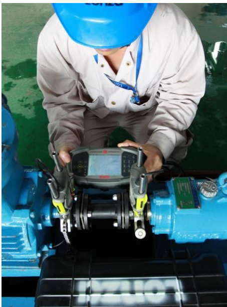
Measuring shaft alignment between motor and pump
