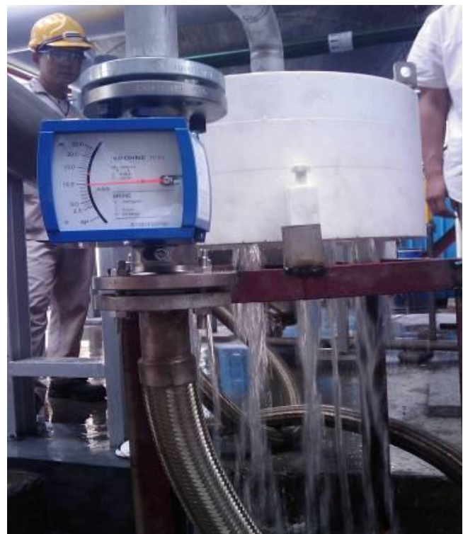
Testing of PTFE distributor for distillation column
